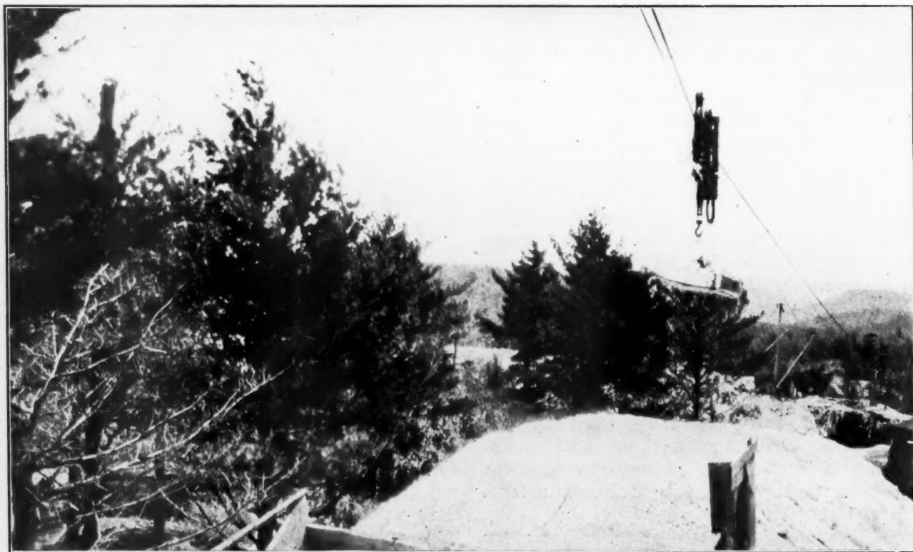
Upper Left—Looking down into the pit with view of one of the mica tunnels. Upper Right—Mica tunnel still full of ice in June. Lower—Load of material approaching the grizzly over the screen at the feldspar sorting plant
